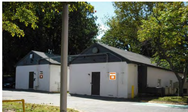
The exterior of Bldgs 22 and 30, two Quonset huts built in the 1960s and used for animal surgery and procedures. Both buildings are slated for demolition.
