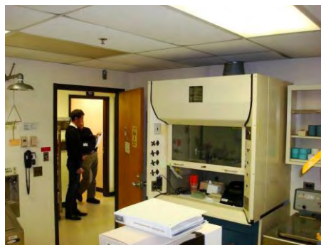
Fume hood blocking laboratory egress, Bldg T-44.
