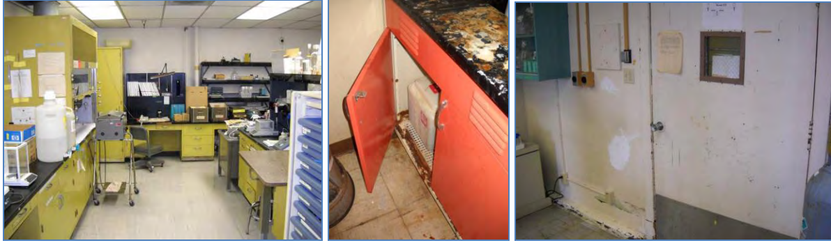
Conditions in Building 113
