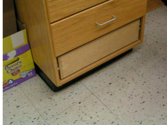
The wood casework in Bldg 35 is not of an appropriate quality for use in research laboratories.
